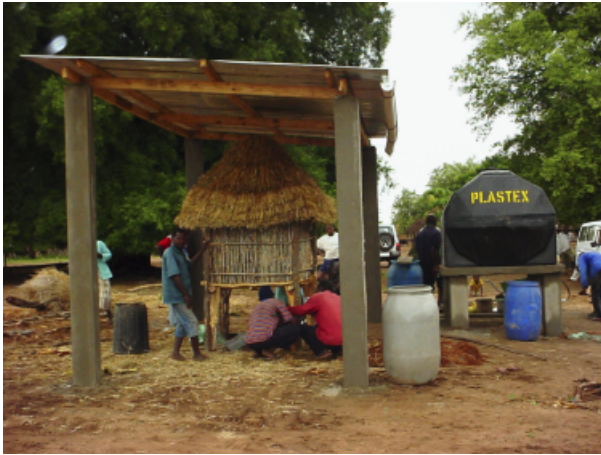
Figure 8 Rainwater harvesting and seed store nearing completion in Matidze.
