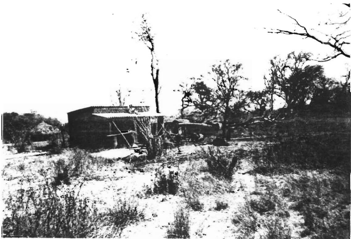
Plate 13: Bush encroachment with the construction of a shop
