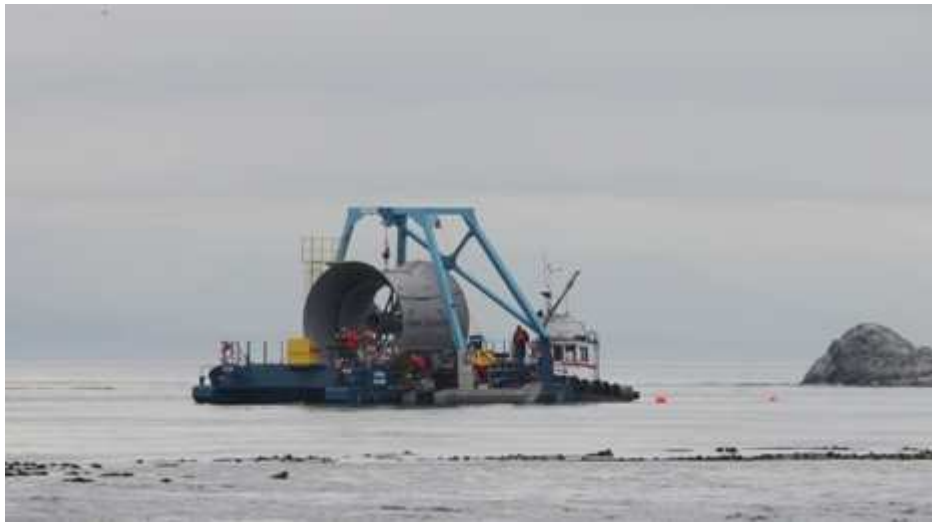
Figure 63 Clean Current turbine during deployment at Race Rocks[87]
