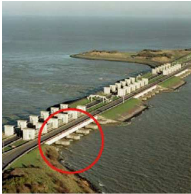
Figure 54 TT Centre Den Oever [70]
