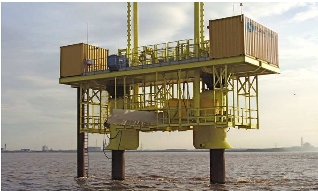
Figure 62 Pulse tidal device installed at the Humber estuary with the blades raised for maintenance [85]
