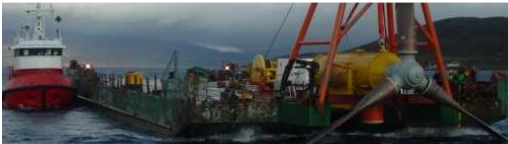
Figure 60 Hammerfest HS300 turbine during deployment at Kvalsund [81]
