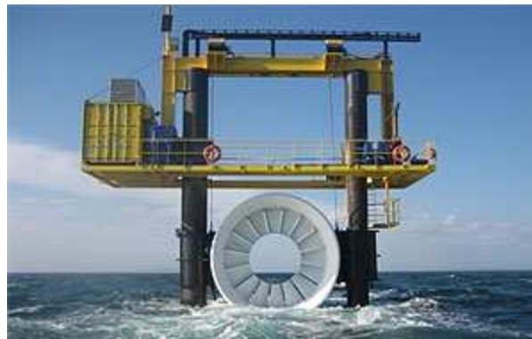
Figure 44 OpenHydro turbine installed at EMEC [48]
