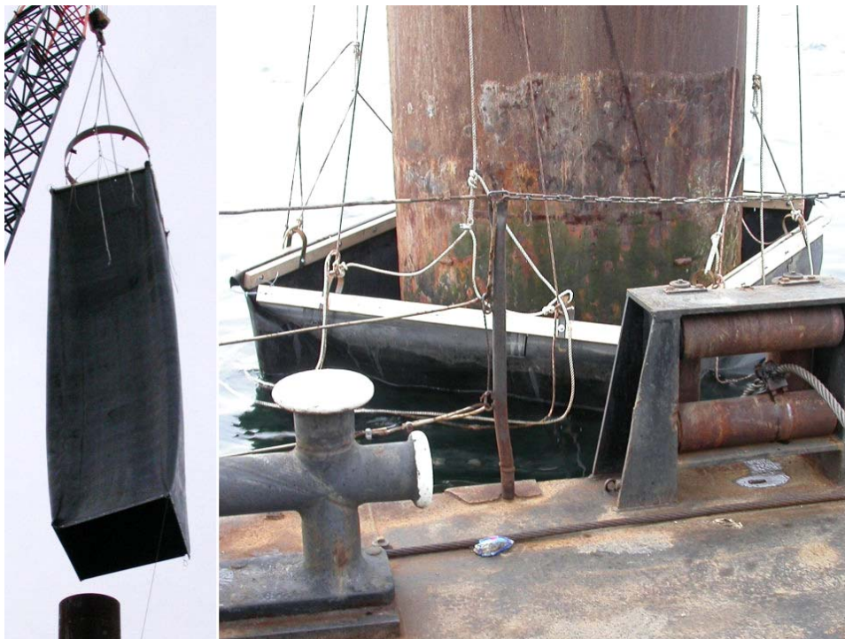
Figure 3-26. Pile sleeve made of 5 mm rubber
