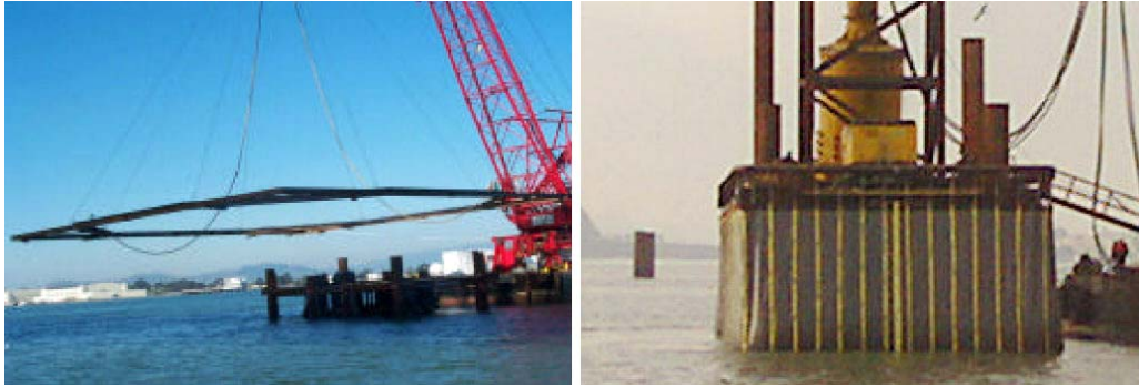
Fig. 3-14. Bubble curtain ring (right) and confined bubble curtain (Reyff 2003)
