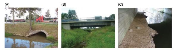
**Figure 35.6** Examples of river otter crossings: (A) unsuitable culvert design with high risk of submersion from flooding, (B) superior design with riparian strips and (C) retrofitted culvert with dry ledge including aquatic entry points for otters. Source: Photographs by N. Klar.
